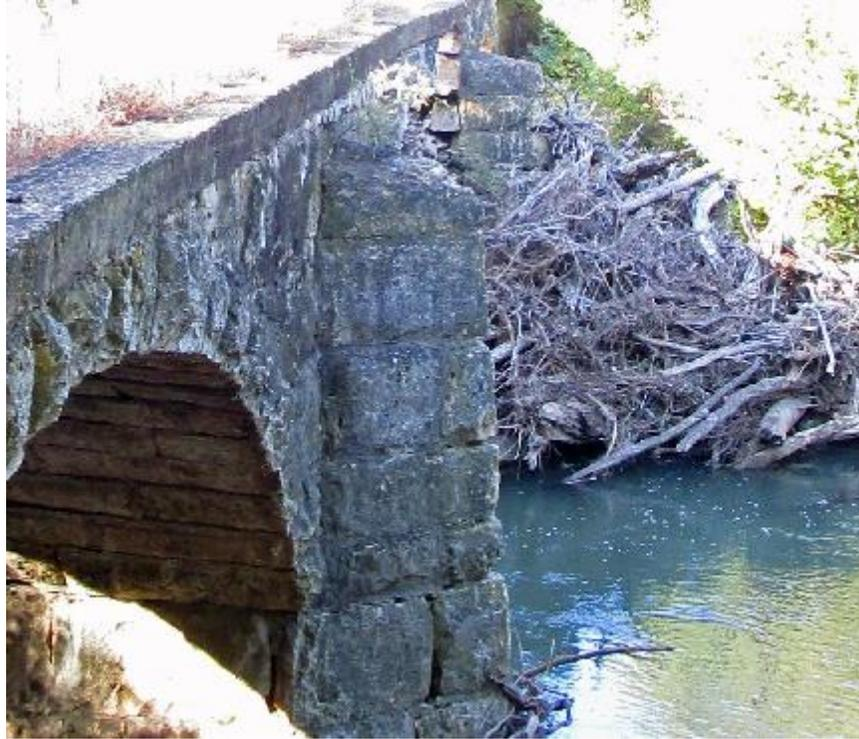
A view of the upstream face of Pudden Bridge, showing loss of masonry of the middle arch (partially obscured by the eastern cutwater). Photo taken on October 20, 2019, facing west.
