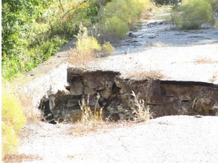
A closeup of the hole in the bridge deck, showing the loss of fill and spandrel walls caused by partial failure of the middle arch.
