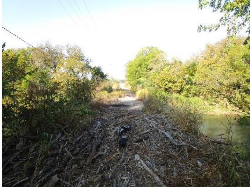
A picture of the overgrown deck of Pudden Bridge taken on October 20, 2019, showing debris left by severe flooding and, towards the far end of the bridge, the hole left in the deck by further collapse of the middle arch. The photo was taken looking west.
