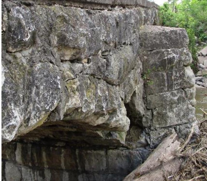
A photograph of the middle arch taken in early May 2019, showing missing arch stones on the upstream face of the arch towards the western pier.
