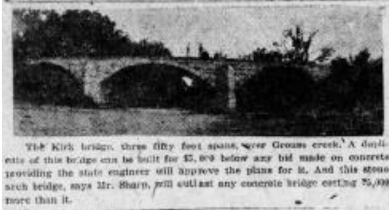
The Kirk bridge, three fifty foot spans, over Grouse creek. A duplicate of this bridge can be built for \$5,000 below any bid made on concrete providing the state engineer will approve the plans for it. And this stone arch bridge, says Mr. Sharp, will outlast any concrete bridge costing \$5,000 more than it.
